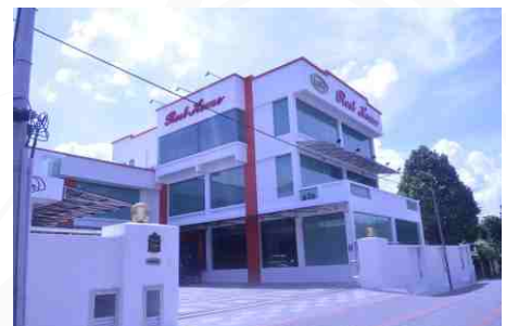
LSH Rest House - Malaysia
