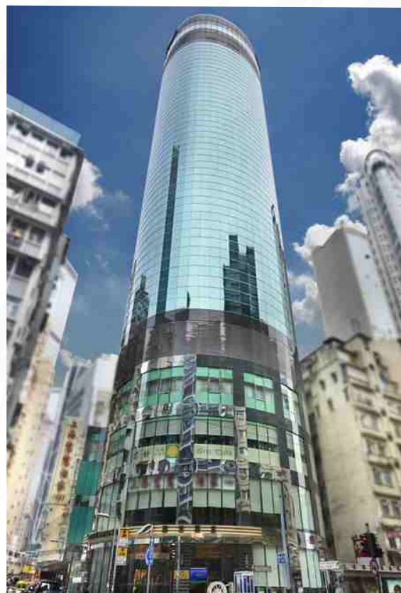
South Pacific Hotel - Hong Kong, China
